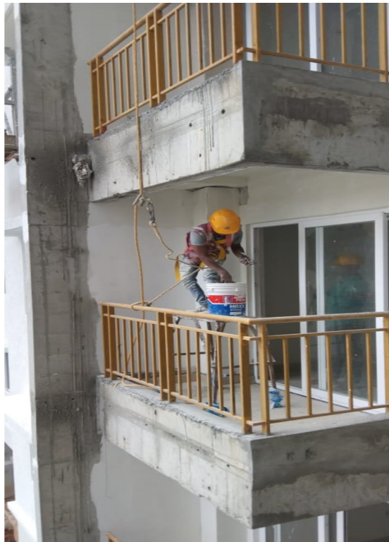
Balcony works execution with life line to arrest fall
